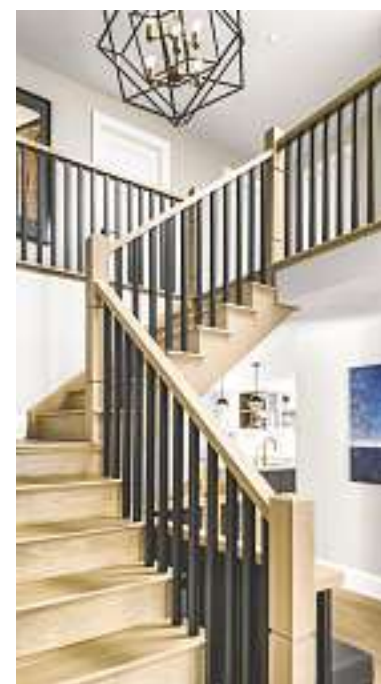
A corner staircase replaces the original circular one and saves space. GILLIAN JACKSON
